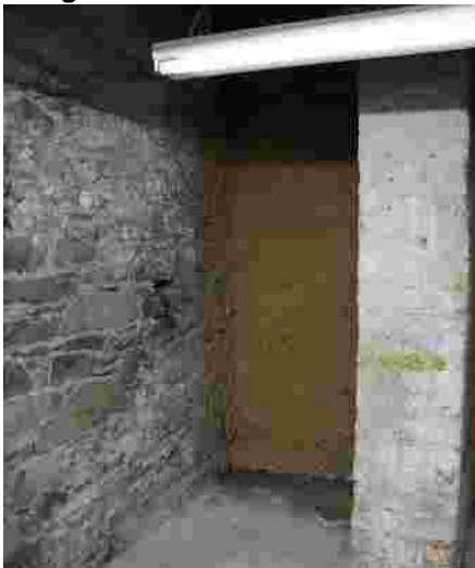
Dungeon/ basement showing a gap in the stone work where shackles once held inmates in solitary confinement April 2008, © Deborah O'Rielly/ HFNL
