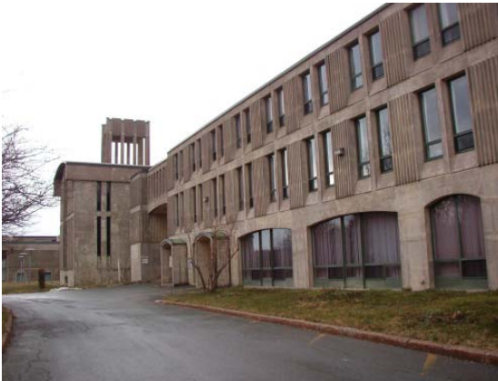
Front façade, south side, Chapel and bell tower at far left
