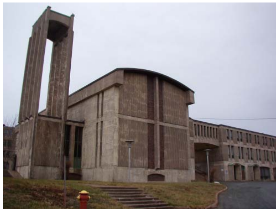
Chapel and bell tower, south facade
